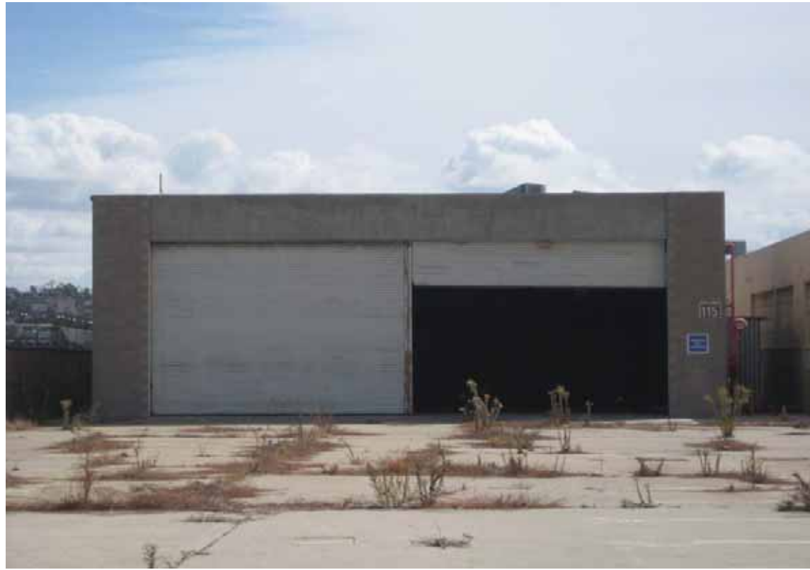
Building 115 - Ancillary Building, West Elevation, San Diego, California, October 2009.
