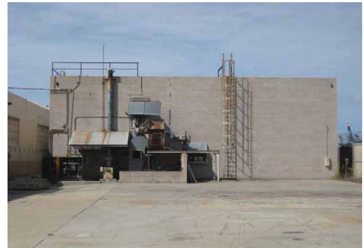
Building 115 - Ancillary Building, East Elevation, San Diego, California, October 2009.
