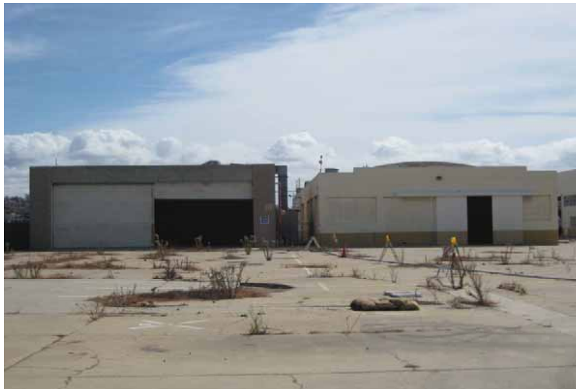
Building 115 - Ancillary Building, West Elevation, San Diego, California, October 2009.
