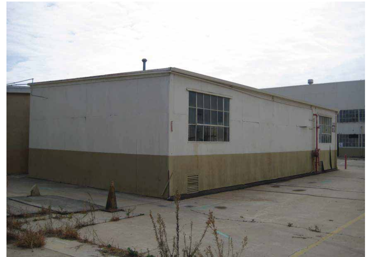
Building 129 - Sandblasting Shed, Northwest Oblique, San Diego, California, October 2009.
