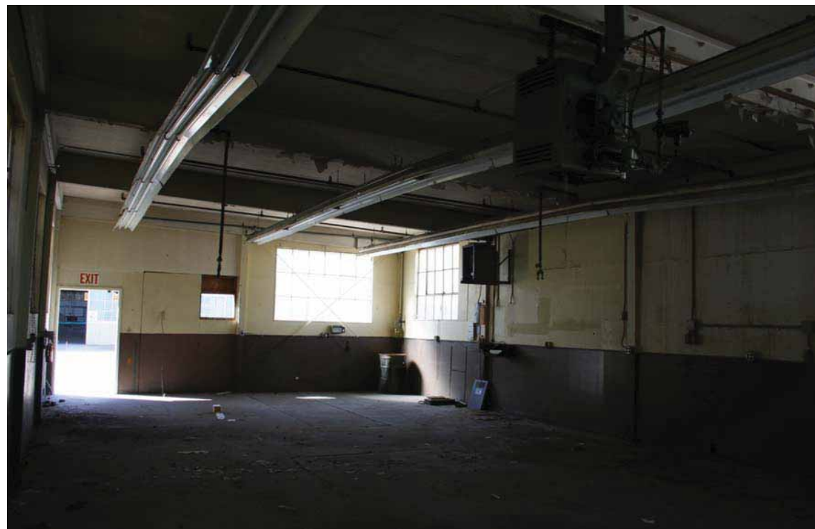
Building 129 - Sandblasting Shed Interior, facing South, San Diego, California, October 2009.
