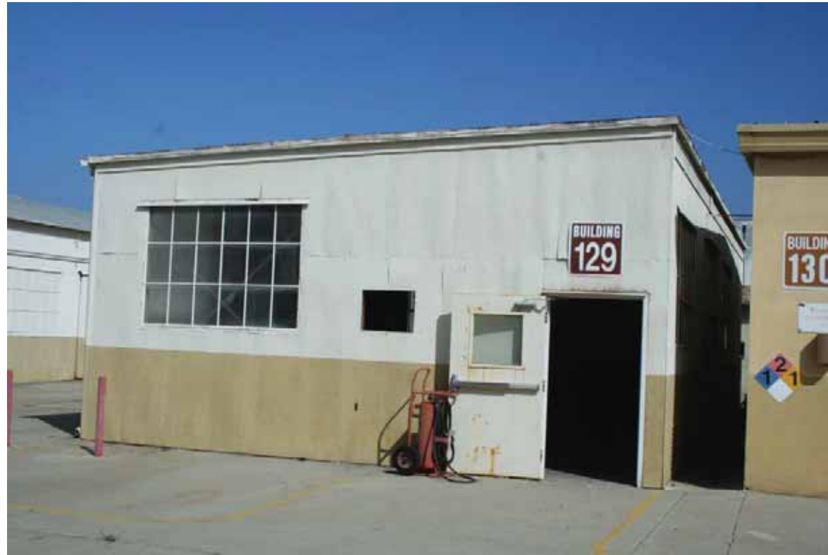
Building 129 - Sandblasting Shed, Southeast Oblique, San Diego, California, October 2009.
