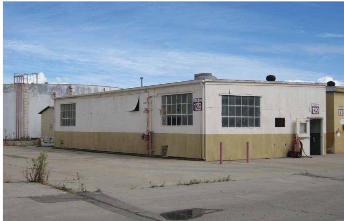
Building 129 - Sandblasting Shed, Southwest Oblique, San Diego, California, October 2009.
