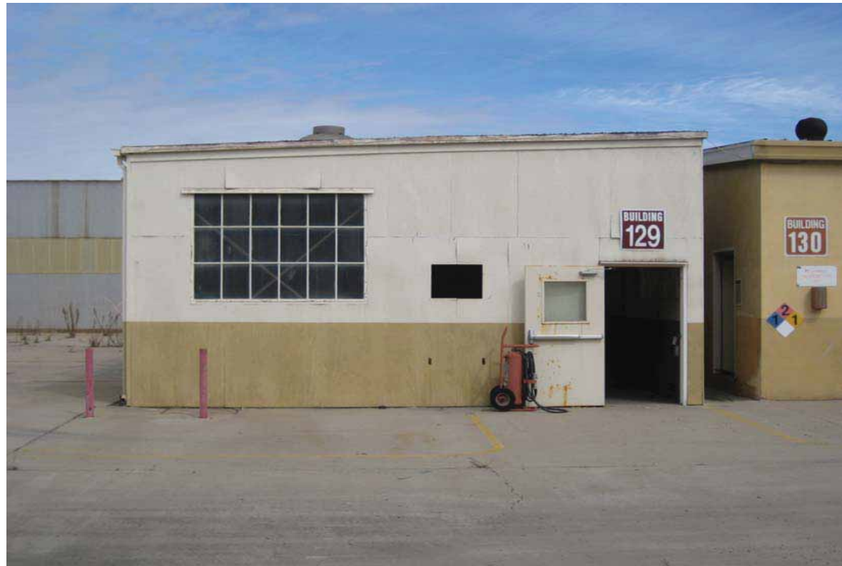
Building 129 - Sandblasting Shed, South Elevation, San Diego, California, October 2009.
