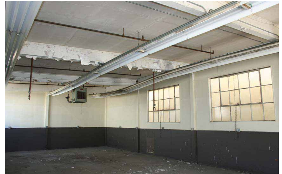
Building 129 - Sandblasting Shed Interior, facing Northeast, San Diego, California, October 2009.
