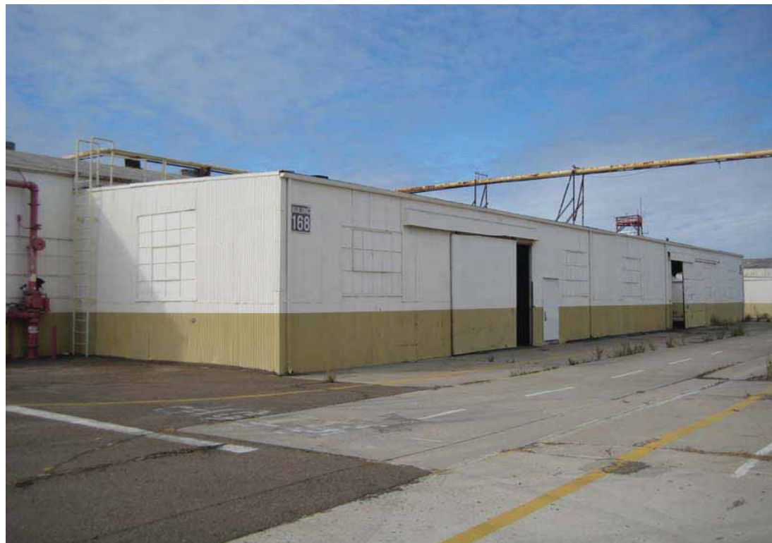
Building 168 – Warehouse Addition Building, Southeast Oblique, San Diego, California, October 2009.
