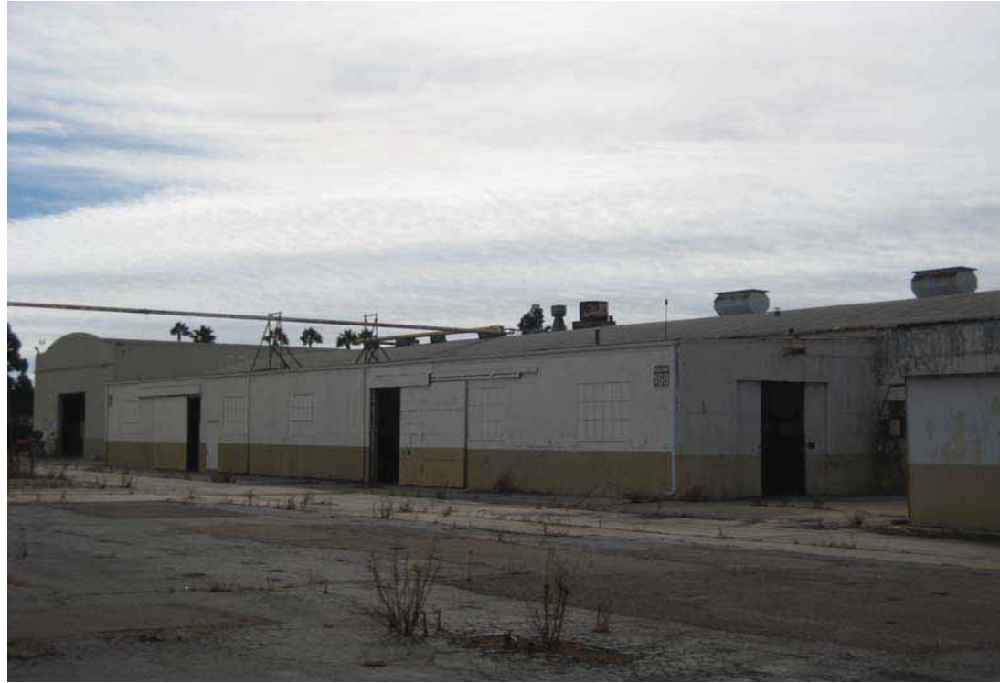
Building 168 – Warehouse Addition Building, Northeast Oblique, San Diego, California, October 2009.
