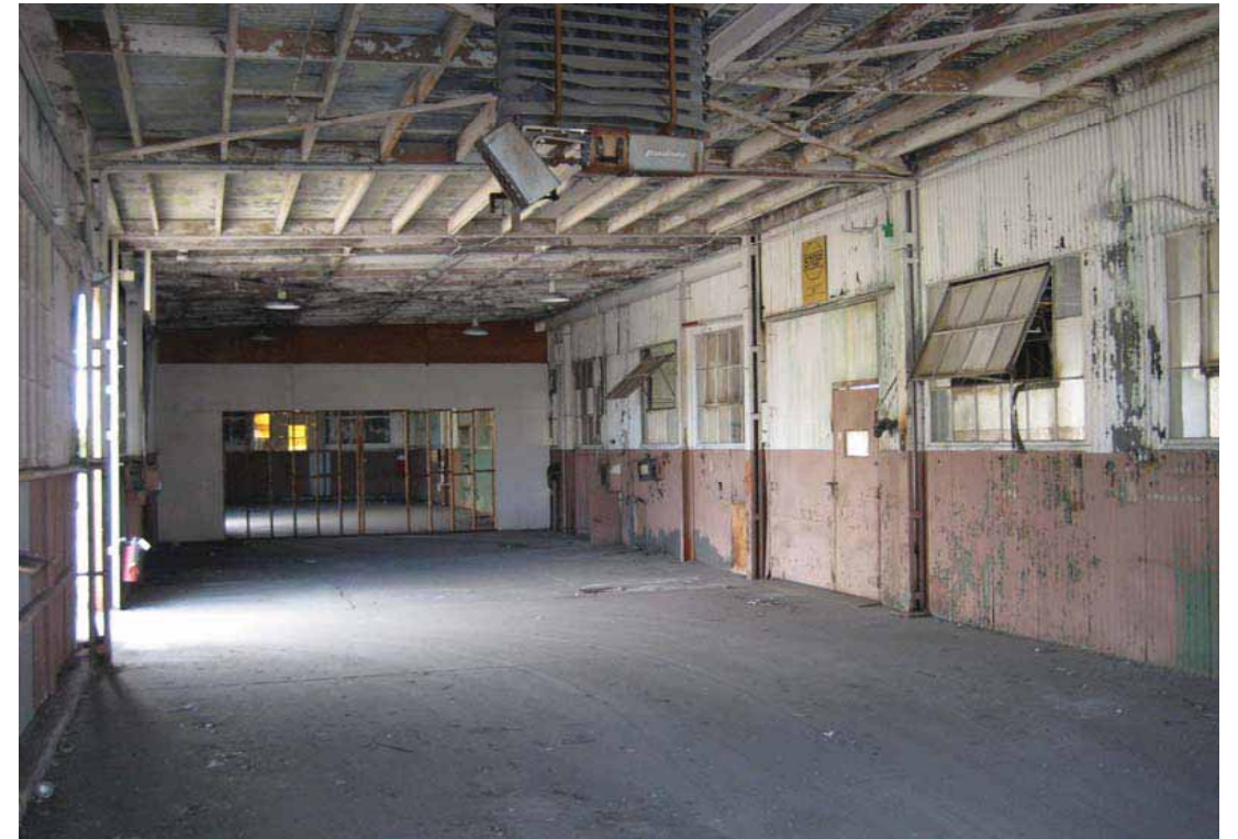
Building 168 – Warehouse Addition Building, Interior Southwest Elevation, San Diego, California, October 2009.
