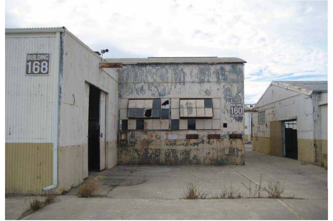
Building 168 – Warehouse Addition Building, South Elevation, San Diego, California, October 2009.
