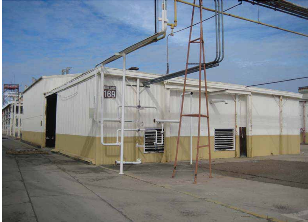
Building 169 - Pattern Staging Building, Southwest Oblique, San Diego, California, October 2009.
