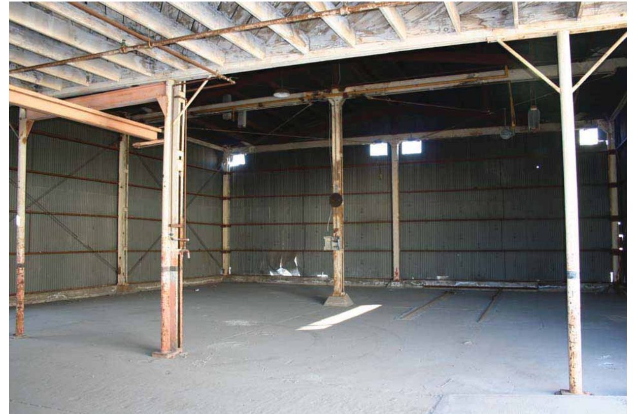
Building 169 - Pattern Staging Building Interior, facing Northwest, San Diego, California, October 2009.
