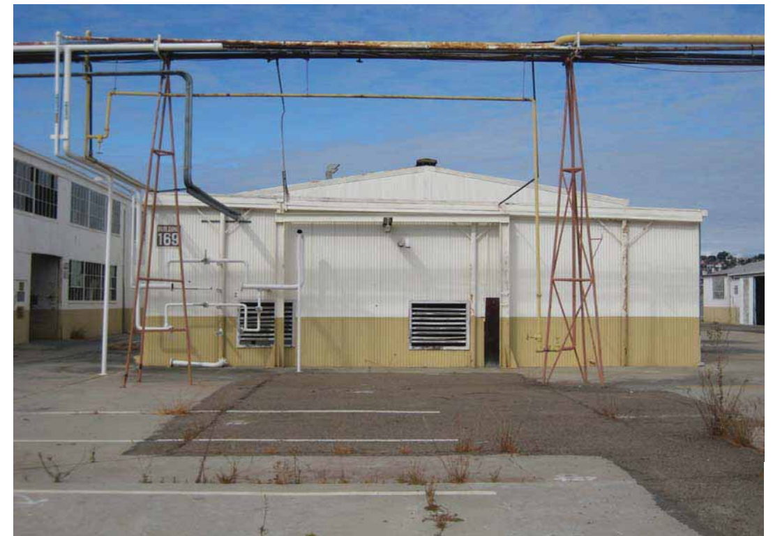
Building 169 - Pattern Staging Building, South Elevation, San Diego, California, October 2009.
