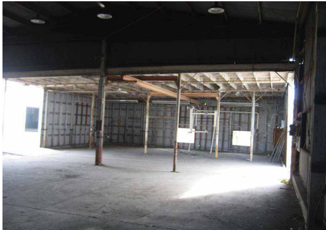
Building 169 - Pattern Staging Building, Interior Northwest Oblique, San Diego, California, October 2009.
