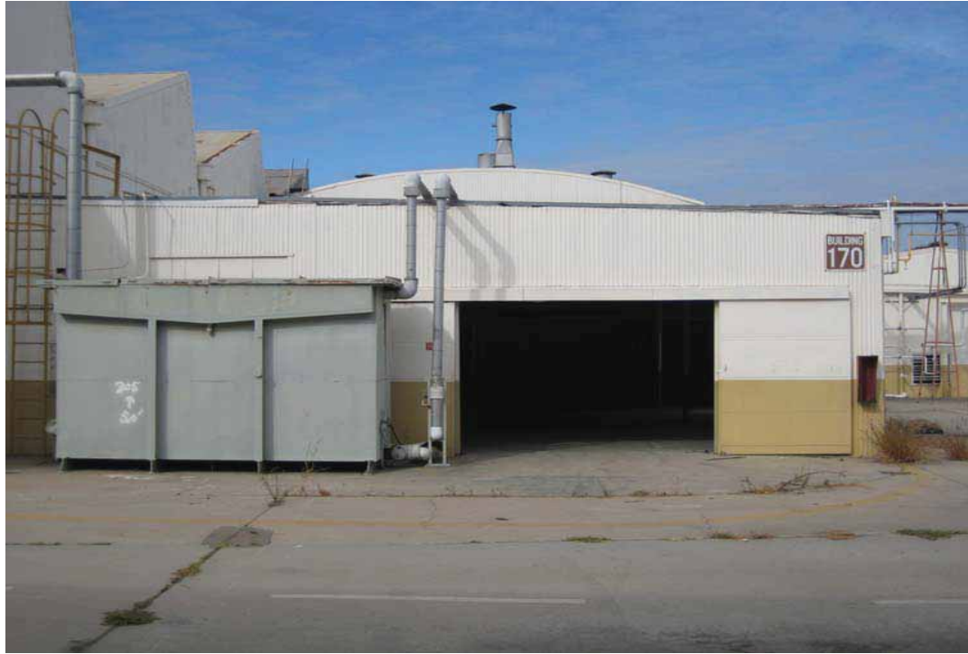
Building 170 - Parts/Drop Hammer Structures, South Elevation, San Diego, California, October 2009.
