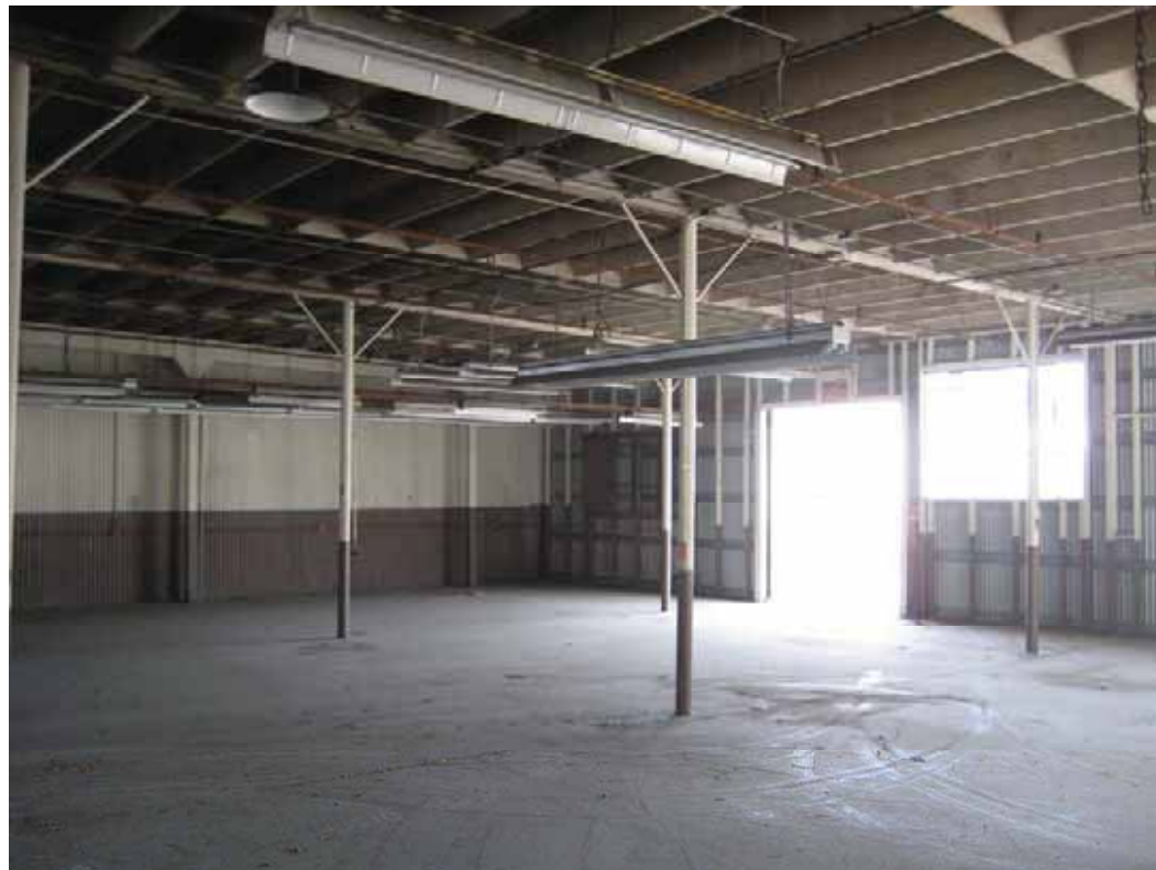
Building 170 - Parts/Drop Hammer Structures, Interior Northeast Elevation, San Diego, California, October 2009.
