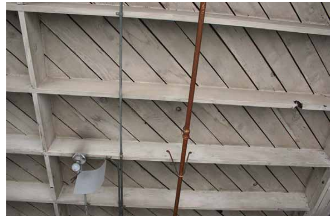
Building 170 - Parts/Drop Hammer Structures Interior, ceiling detail, San Diego, California, October 2009.
