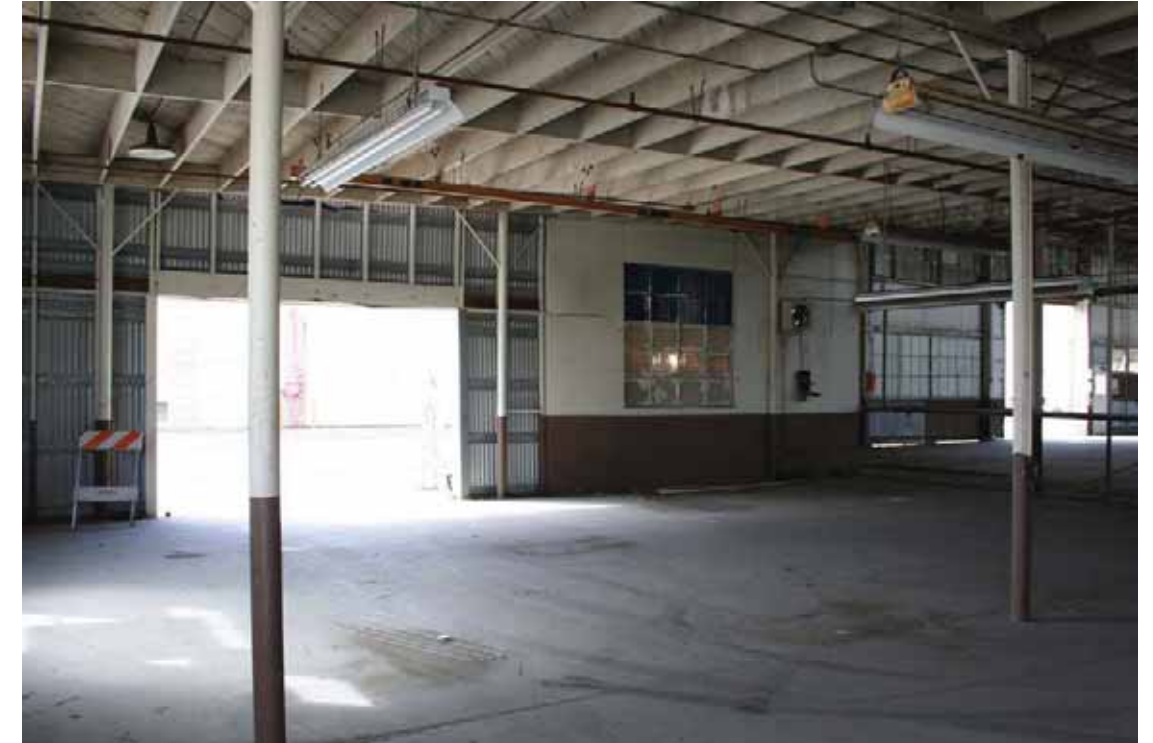
Building 170 - Parts/Drop Hammer Structures Interior, facing Southwest, San Diego, California, October 2009.
