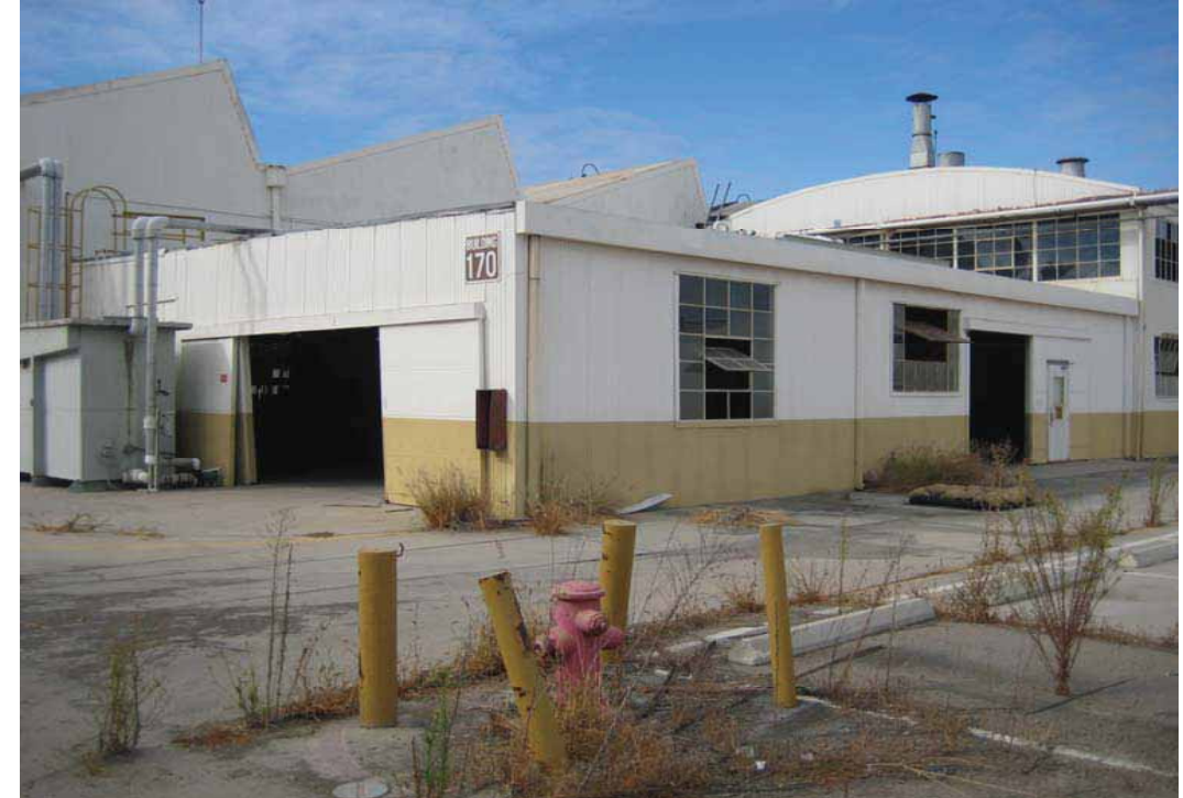
Building 170 - Parts/Drop Hammer Structures, Southwest Oblique, San Diego, California, October 2009.
