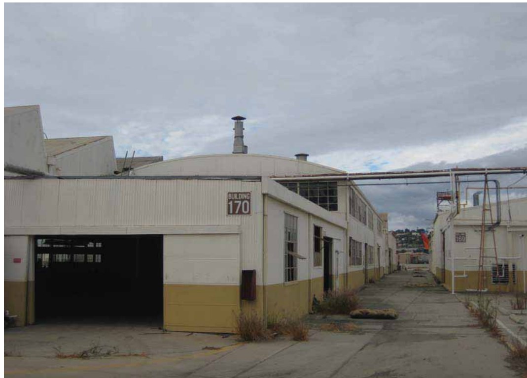
Building 170 - Parts/Drop Hammer Structures, Southeast Elevation, San Diego, California, October 2009.
