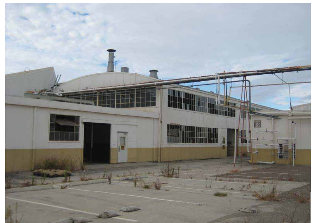
Building 170 - Parts/Drop Hammer Structures, Northwest Oblique, San Diego, California, October 2009.
