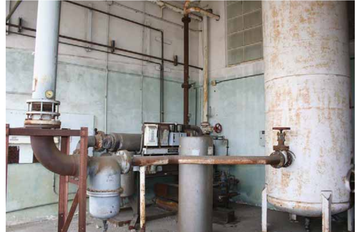
Building 230 - Interior, East Wall facing East, San Diego, California, October 2009.
