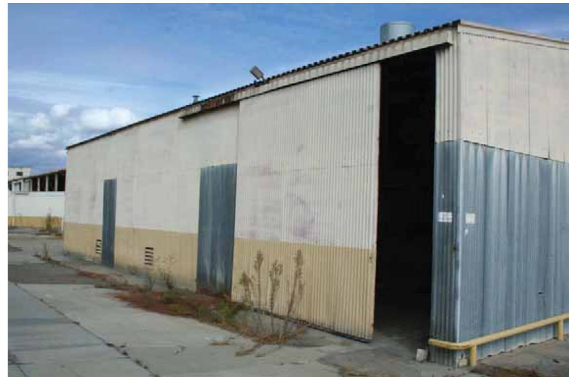
Building 513 - Ancillary Building Associated With Building 156, West Elevation, San Diego, California, October 2009.
